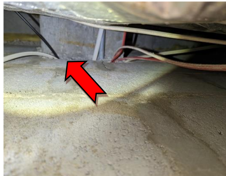
6. Representative photograph of low risk, good condition assumed asbestos-containing fire proofing.
