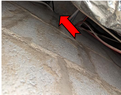
4. Representative photograph of low risk, good condition assumed asbestos-containing fire proofing.
