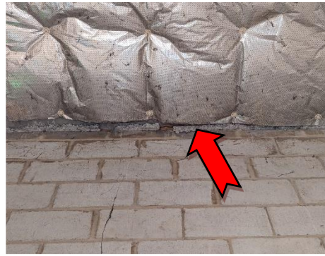
2. Representative photograph of high risk, poor condition, structurally unstable assumed asbestos-containing fire proofing.
