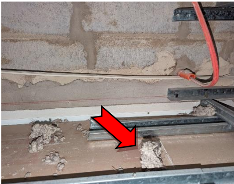
5. Representative photograph of high risk, poor condition, assumed asbestos-containing fire proofing debris.
